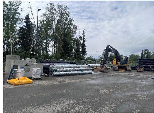
Material and equipment storage
