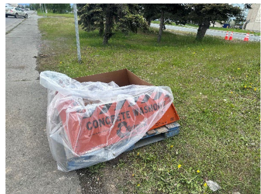
Lined concrete washout
