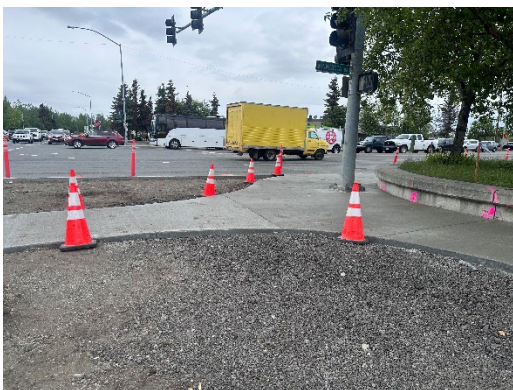
New concrete at Benson and Minnesota
