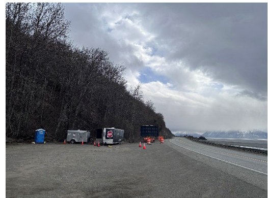
Flagging contractor staging area and sign
