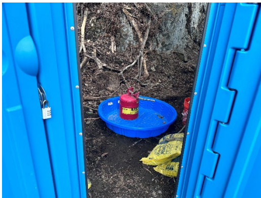
Secondary containment fuel storage
